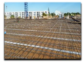
6 Field-placed reinforcing steel is installed.
