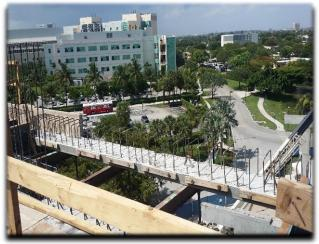
2 Soffit Beams are lowered into place, and shoring or scaffolding is erected to receive the precast/ prestressed joists.
