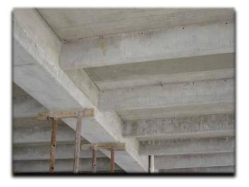
8 After concrete has cured sufficiently, pins, angles, purlins and plywood sheets are removed from the underside of the composite slab system.
