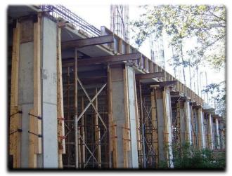
1 Shoring is set between columns to Support the precast Soffit Beams.
