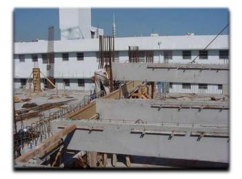
3 Slotted Soffit Beam side forms are attached and joists are then lowered into the slots in the beam form.
