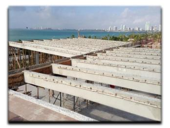
4 Steel pins are inserted in joists and angles are attached to support deck formwork. This hardware may be installed before the joist is set to further facilitate erection.
