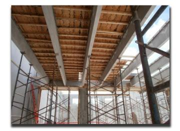
5 Slab formwork material consisting of purlins and plywood decking are placed on these angles.
