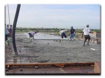
7 Concrete is poured, screeded, floated, and troweled to the required finish.
